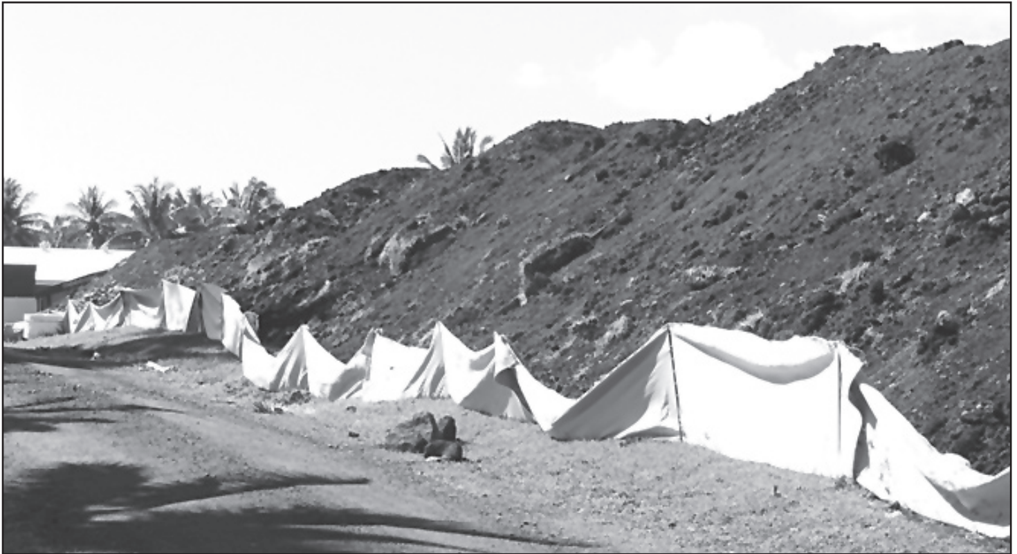
Use of silt fences on the construction of the multi-complex by T&M contractors
